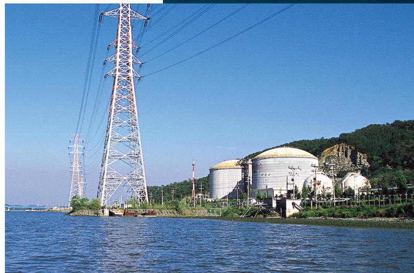
↑ SK Gas began to solidify its position as a major LPG player when it built the Pyeongtaek Terminals in 1999. The refrigerated butane tanks at the Pyeongtaek Terminals constituted the first project of its kind in Korea.
