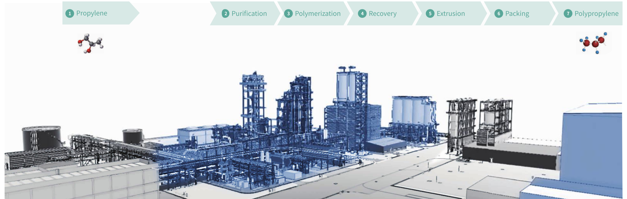
Production process of PP in Ulsan
