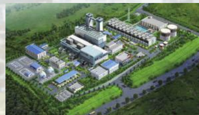
LPG/LNG combined cycle power plant
